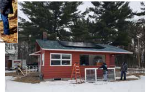
Duralum Building Center, Inc. installing new windows at NCCT's office.
